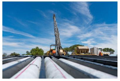
A parallel programme, totalling 1,415m of geotechnical core drilling across 8 holes was completed in late January 2023. The programme was designed to provide additional geotechnical information for pit wall stability studies and minimise waste stripping by optimising pit wall angles. The recommendations resulting from the programme will be incorporated into the pit designs for the reserve Bankable estimation and Feasibility Study.
